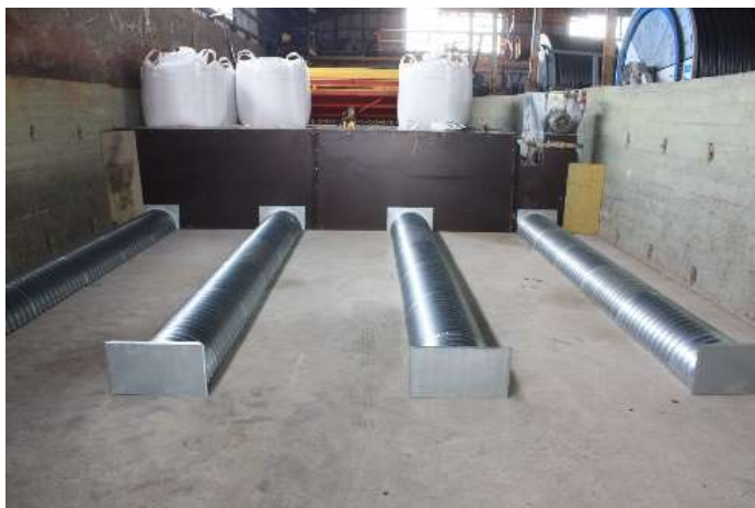
Figure 2. Facilities for aeration storage or drying.
